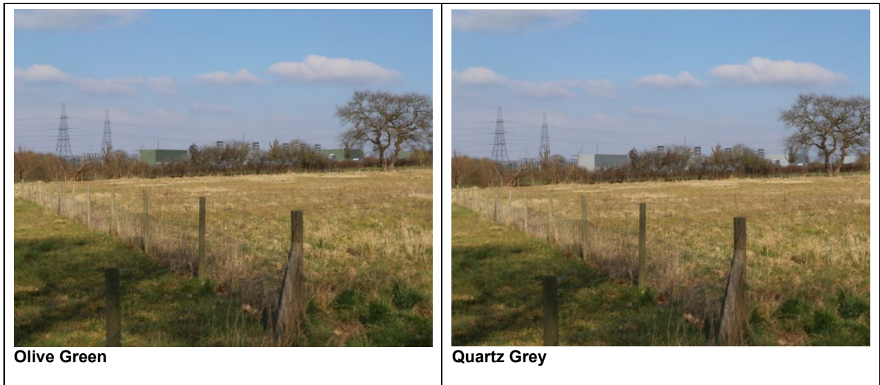
Plate 4.4 Viewpoint 2 Extract: Example of different colour treatments for substation buildings (Document Number ExA.AS-30.D8.V1)
